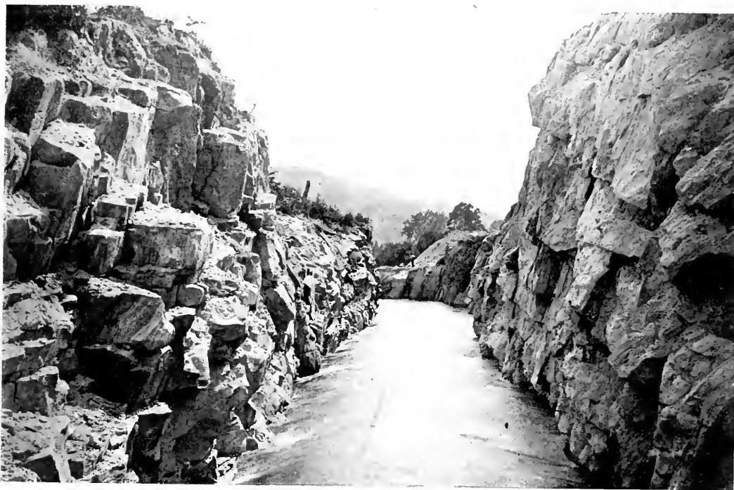
FIG. 1.—WATER IN THE DEEP CUT OF THE CANAL.
